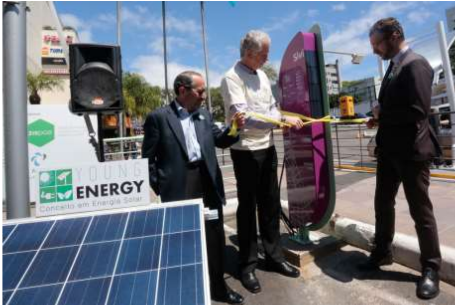
Solar Recharge Station at Shopping Mall
