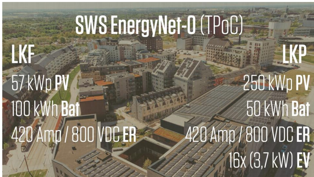
Fig. 9. The official full name of the installation: SWS (Solar-Wind-Storage) EnergyNet System – 0, this illustration shows the capabilities on each side, and the connection.
